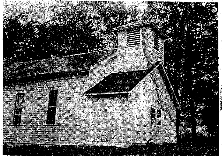
BUILT IN 1874 WAS the New Hope Baptist Church on State Route 554 near Rio Grande. The church sometimes was referred to as the Harris Colored Baptist Church because it was close to Harrisburg, but there's no assurance that this was ever an official name. In 1874 a Republican rally was held here as well as at Providence Baptist (also called Buck Ridge).
